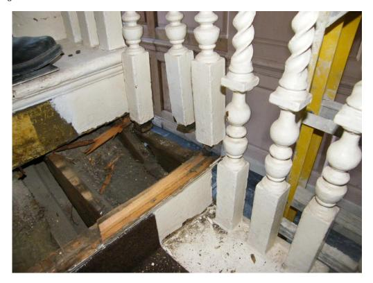
There were four treads on the first two flights where the single piece softwood board has split laterally. The defect has occurred as the irregular triangular blocking pieces have dropped slightly due to historic deflection in the framing below.
