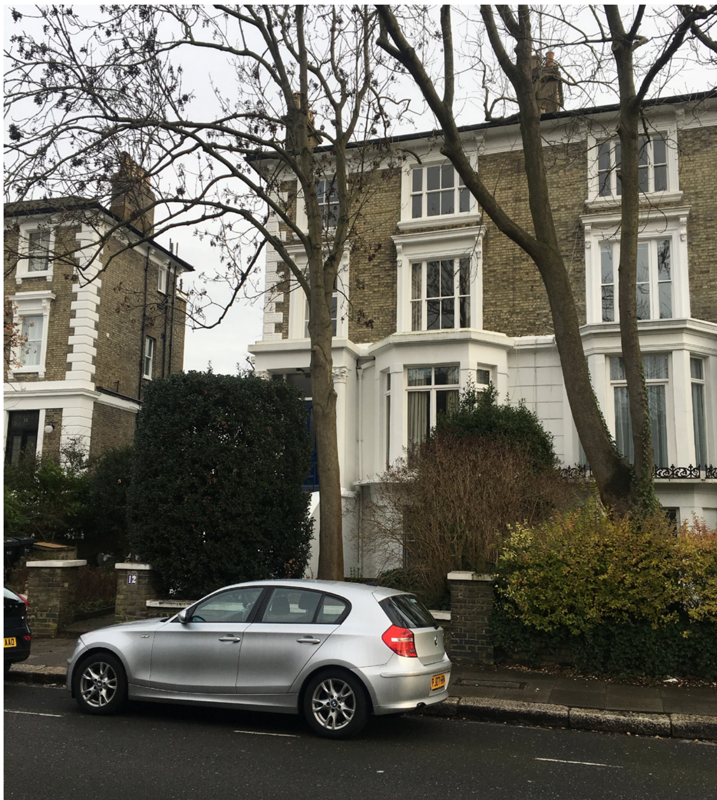
Front elevation of 12 Lawn Road
