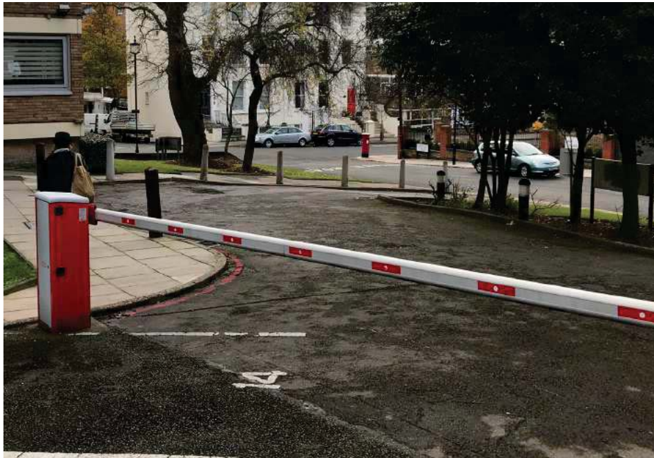
Existing Hard Landscaping
