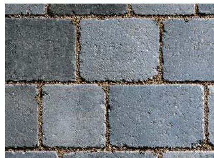
03 Permeable Block Paving
