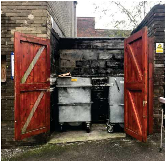
Existing waste / recycling storage unit servicing Barrie House
