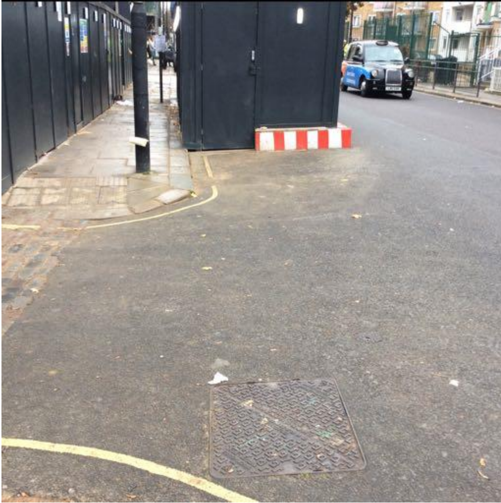
road outside - bayham street
