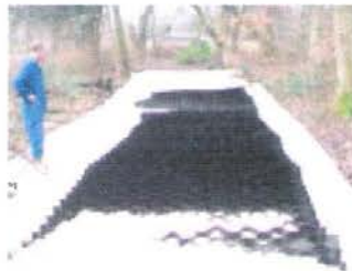
Installation of the CellWeb™ system.
