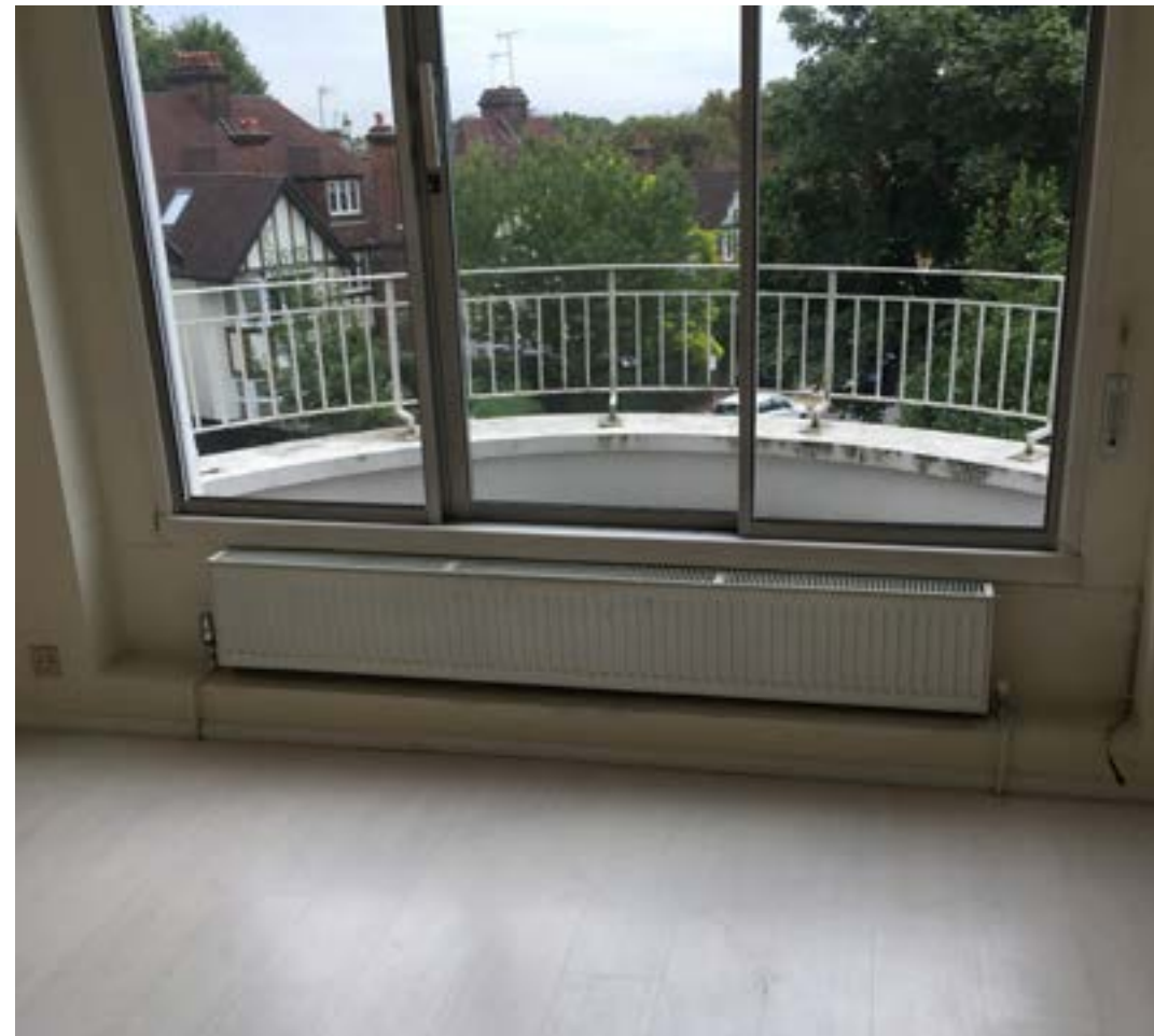
Fig.4. Existing aluminium window fitted within original double door opening.
