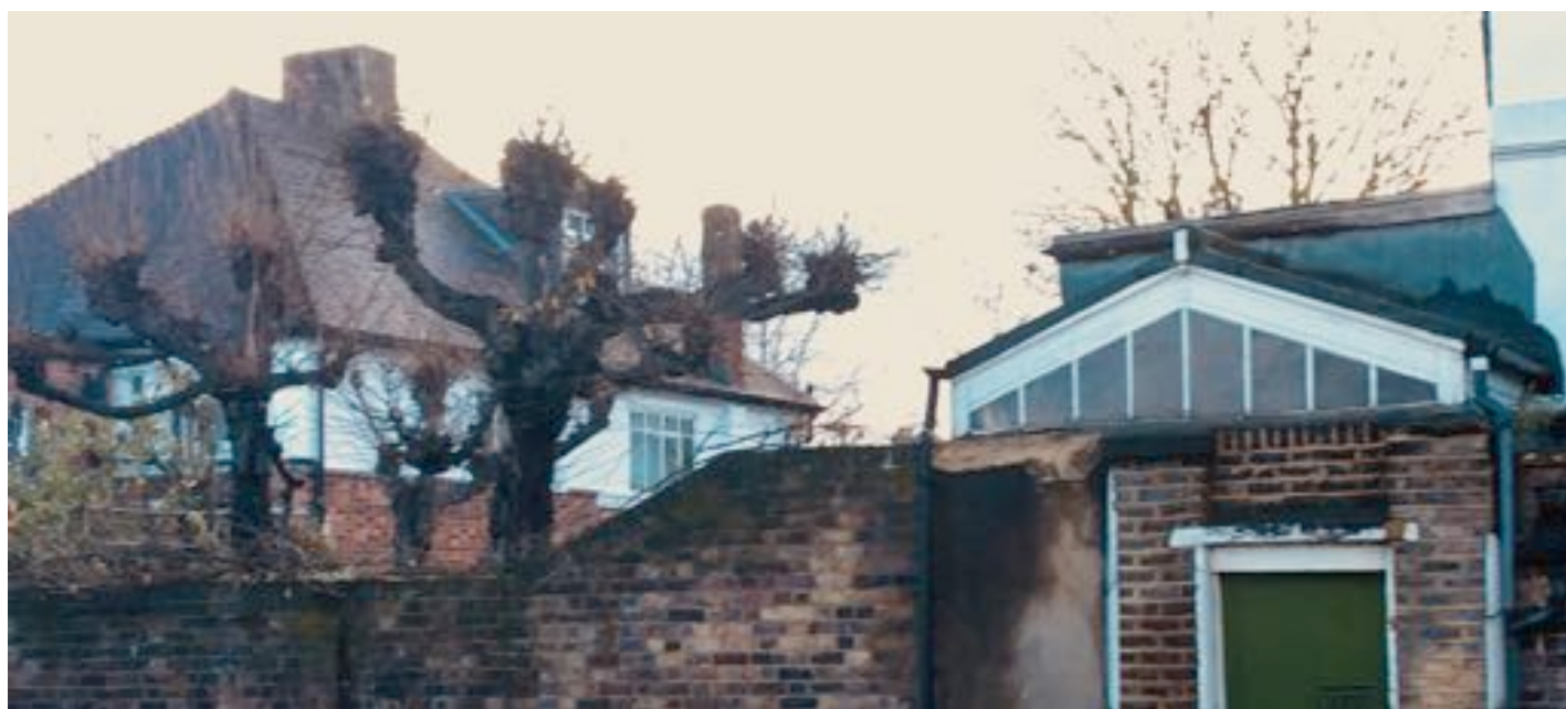
WINODWS AND ROOFS ABOVE STREET BOUNDARY WALL
