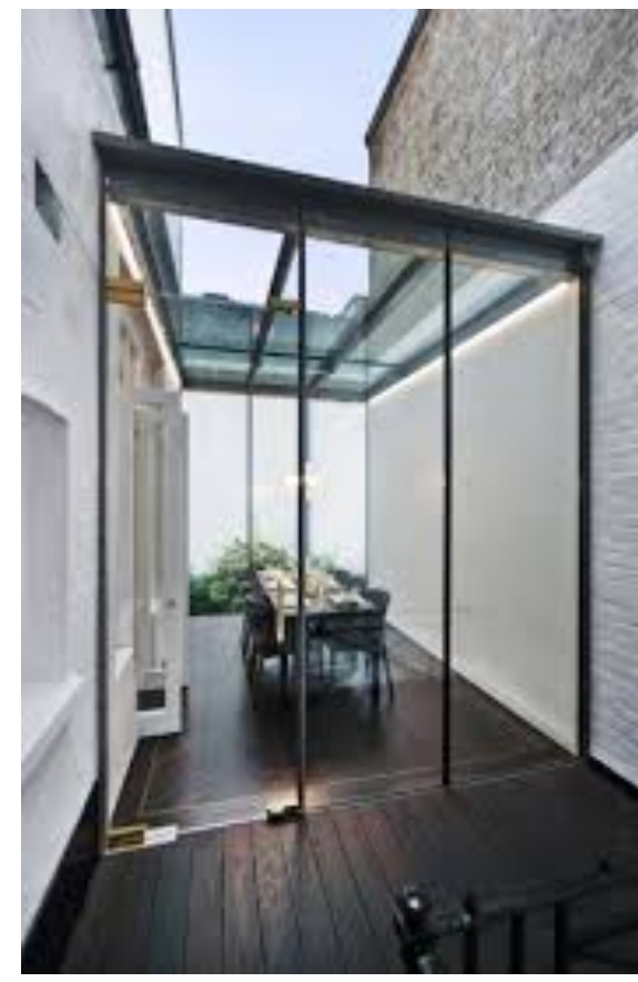
EDGE CHANNEL & BLACK FRAME GLAZED ROOF
