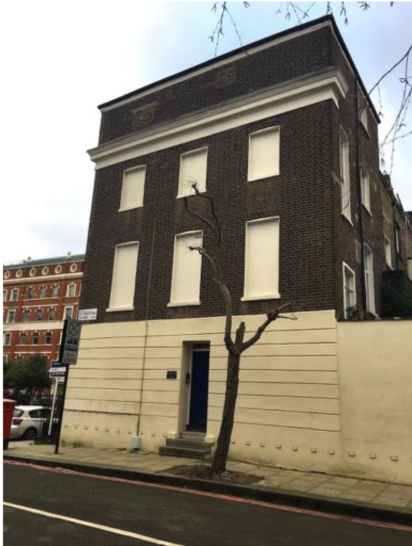
93 CAMDEN ST ENTRANCE ON ST MARTINS CLOSE
