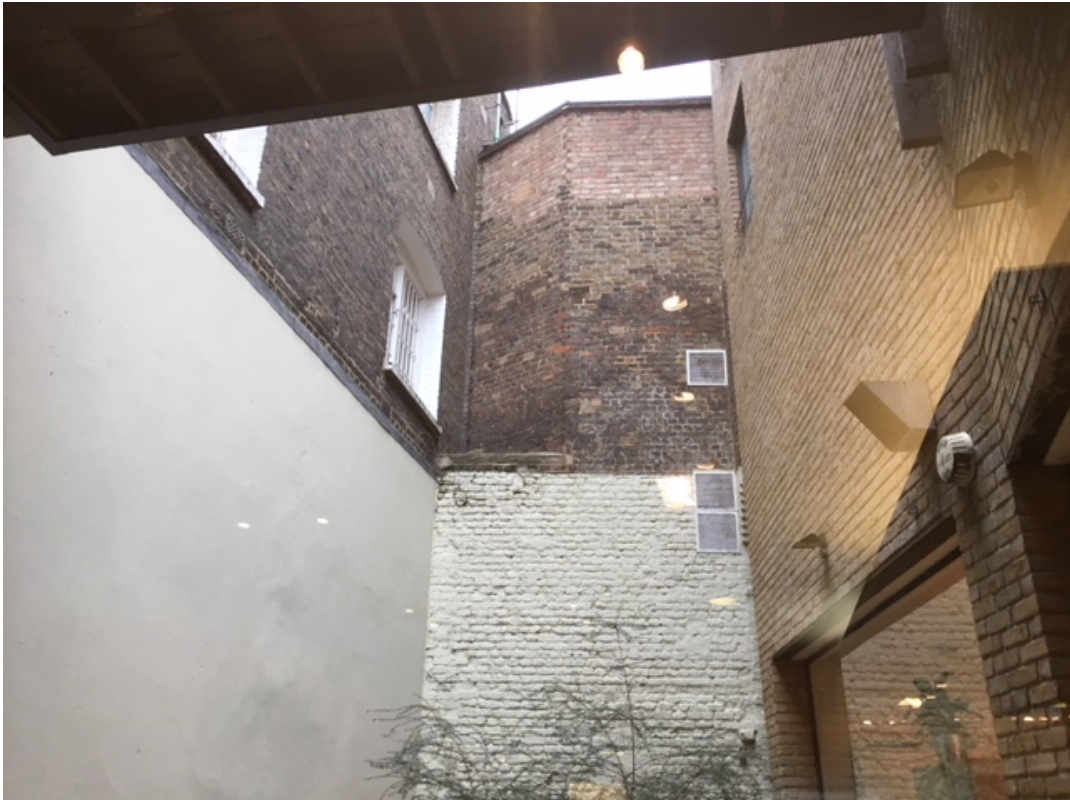
5. Looking towards courtyard from existing shop floor
