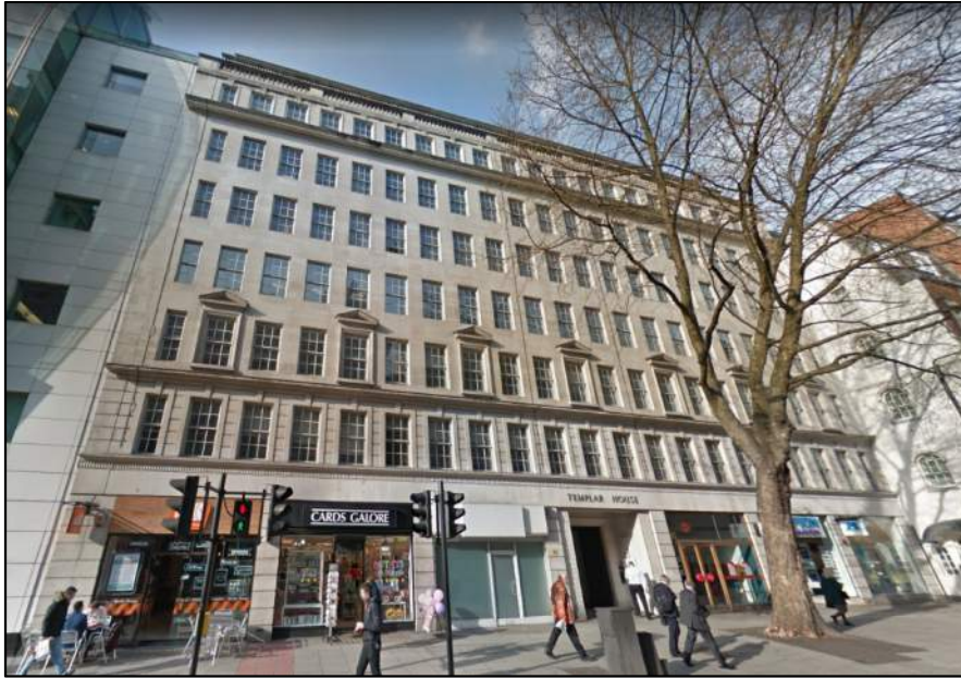
Figure 3 – Street view of Templar House on High Holborn 1
