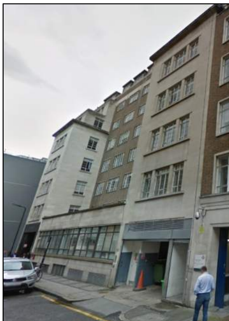
Figure 6 – Street view of 28-34 Eagle Street 1
