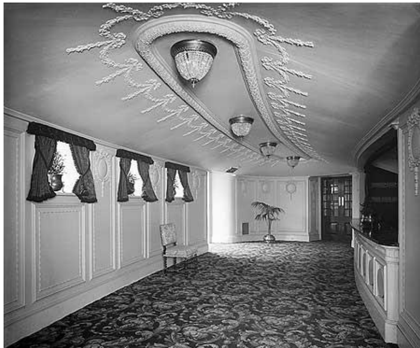
Ground Floor Ambulatory [1911] Note Location of Bar Since Removed
