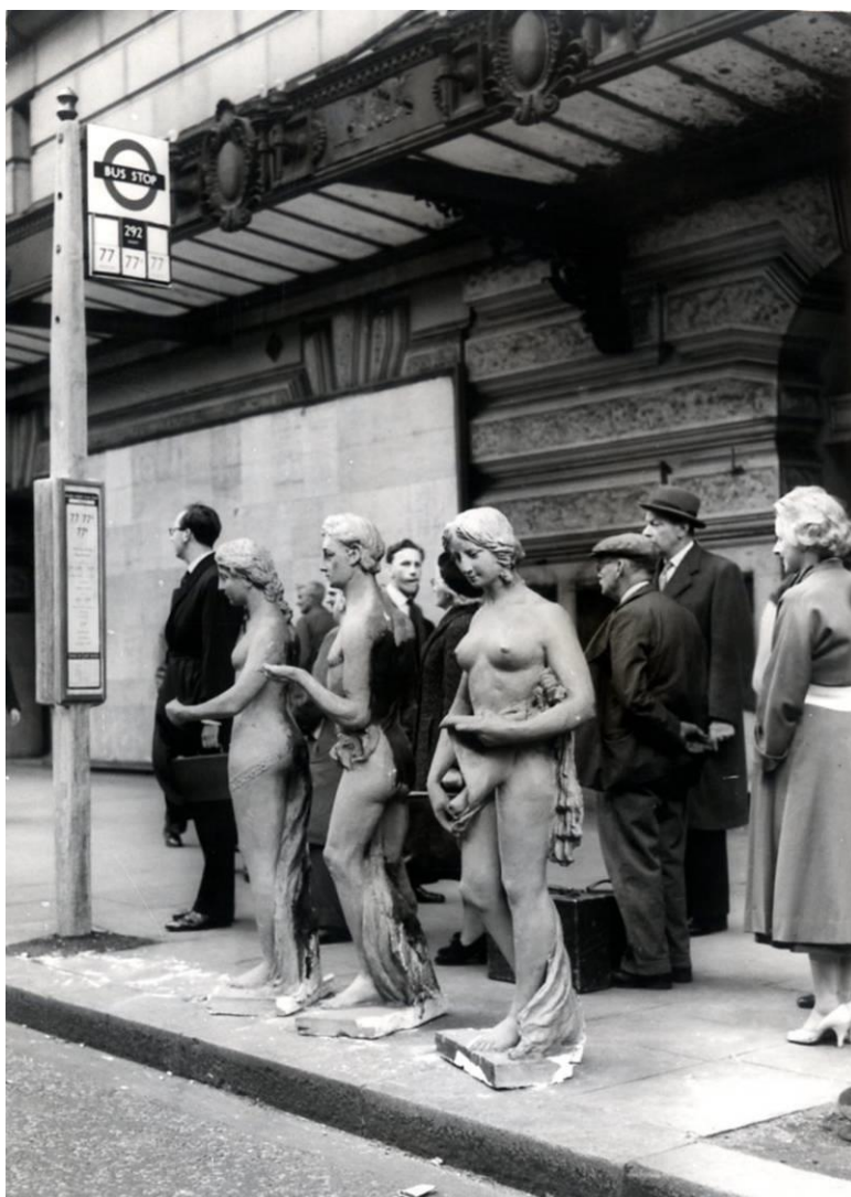
London Opera House – Rudge's Statues Removed from the Parapet Prior to Demolition, November 1957 [theatresearch archive]
