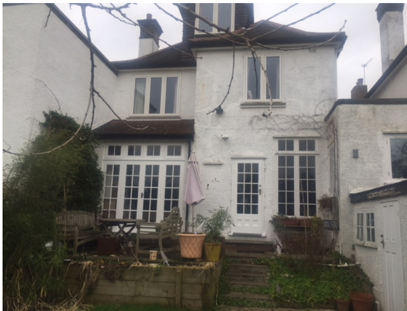
Photo 4: Rear elevation (lower fenestration to be replaced with French doors)
