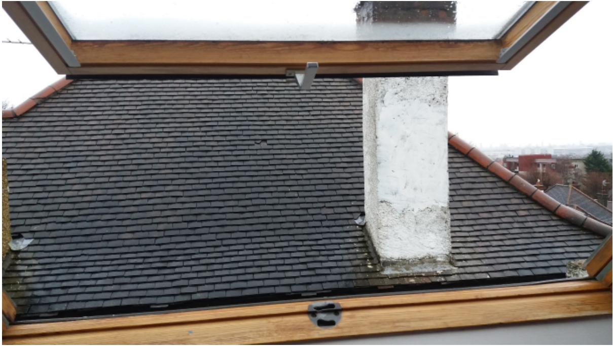
Photo 5: View (from existing velux) of approximate overlook from proposed dormer roof extension
