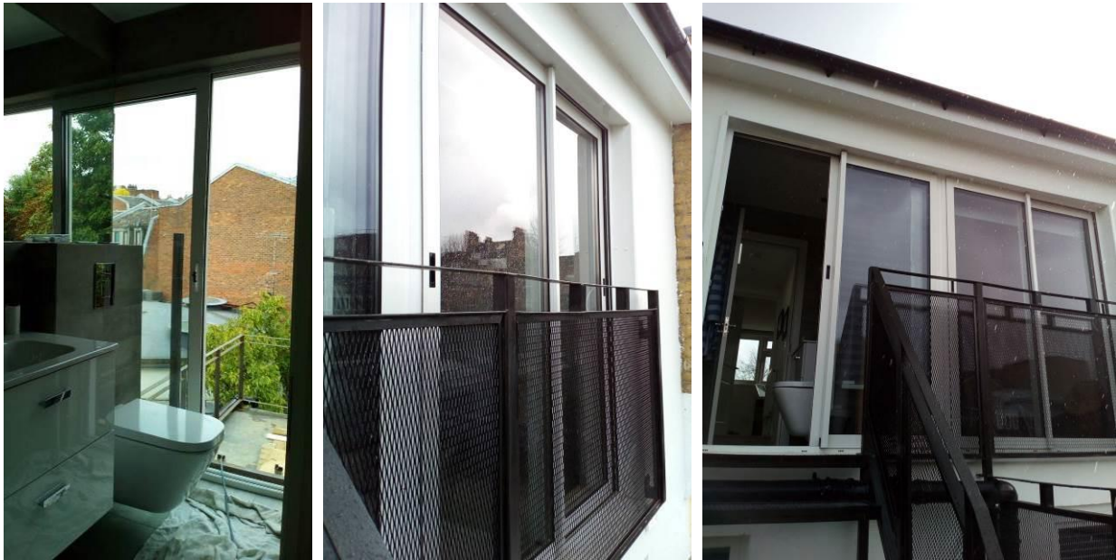
Figures 9, 10, 11. View of dormer from flat roof (figure 9 during construction). Steps and railings on the north side to be removed. Dormer doors balustrade to be kept with the design that matches the railings.
