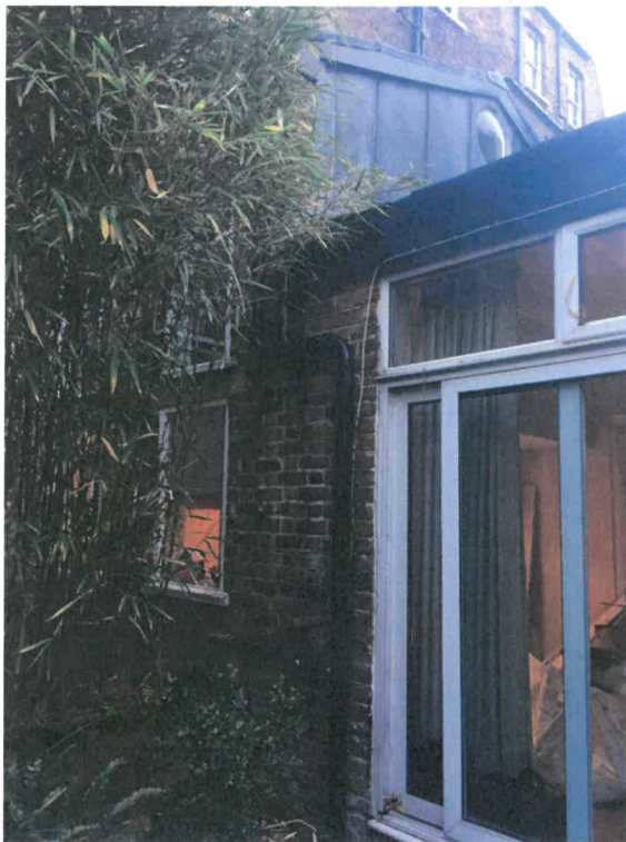
13. Windows to side wall upper level
