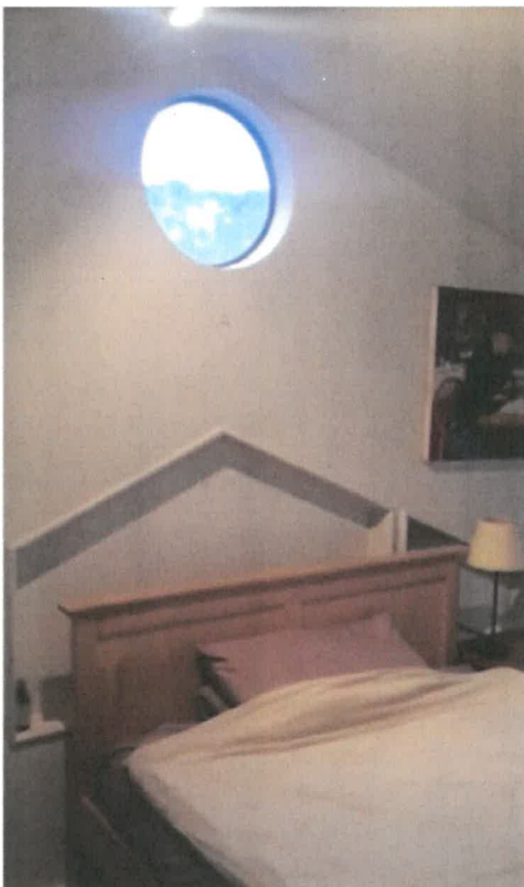
10. Master Bedroom – First Floor Showing Porthole window and painted over internal window.
