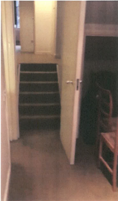
9. Steps From Living Room up to Hallway
