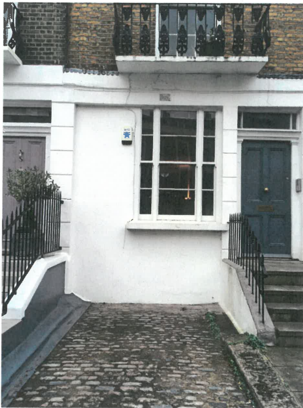
1. Bedroom 2 window showing 'infilled' rote to rear.
