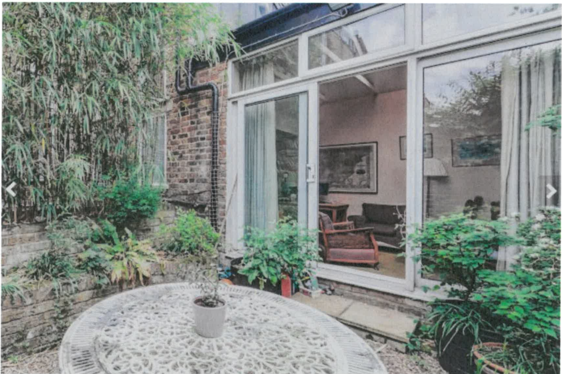
12. External Windows / Doors to Living Room.
