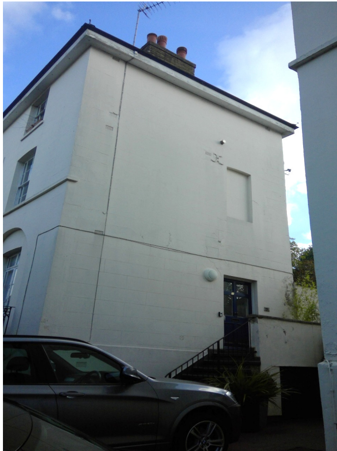
98 Fortess Road – Side elevation and front entrance
