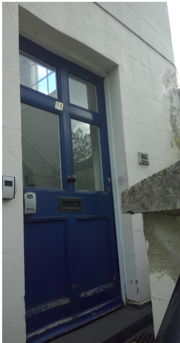
98 Fortess Road- Door Detail
