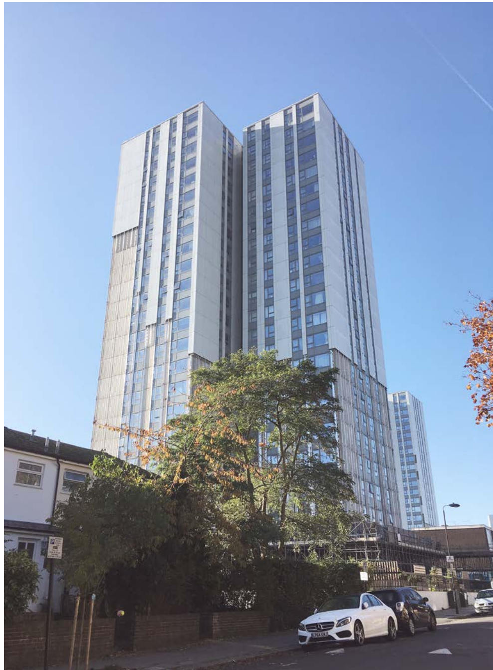
V10 - Existing Dorney Tower, mid cladding removal (from Fellows Rd)
