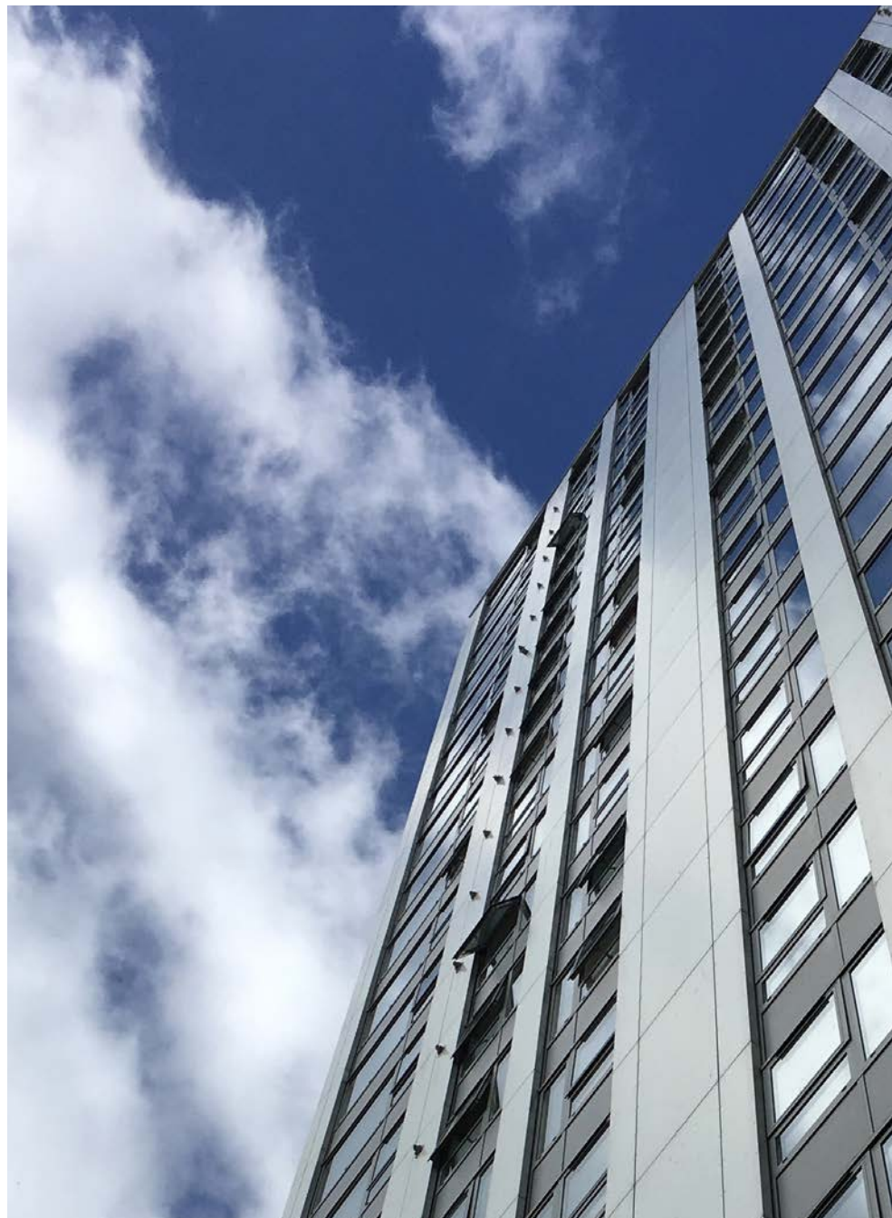
Existing Taplow Tower
