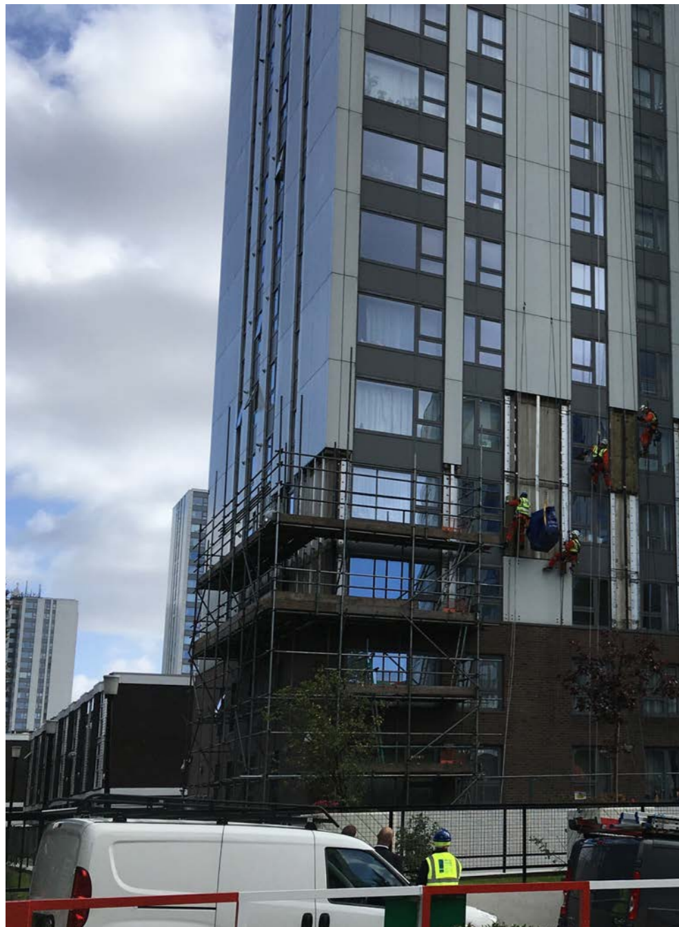
Initial Cladding Removal Works
