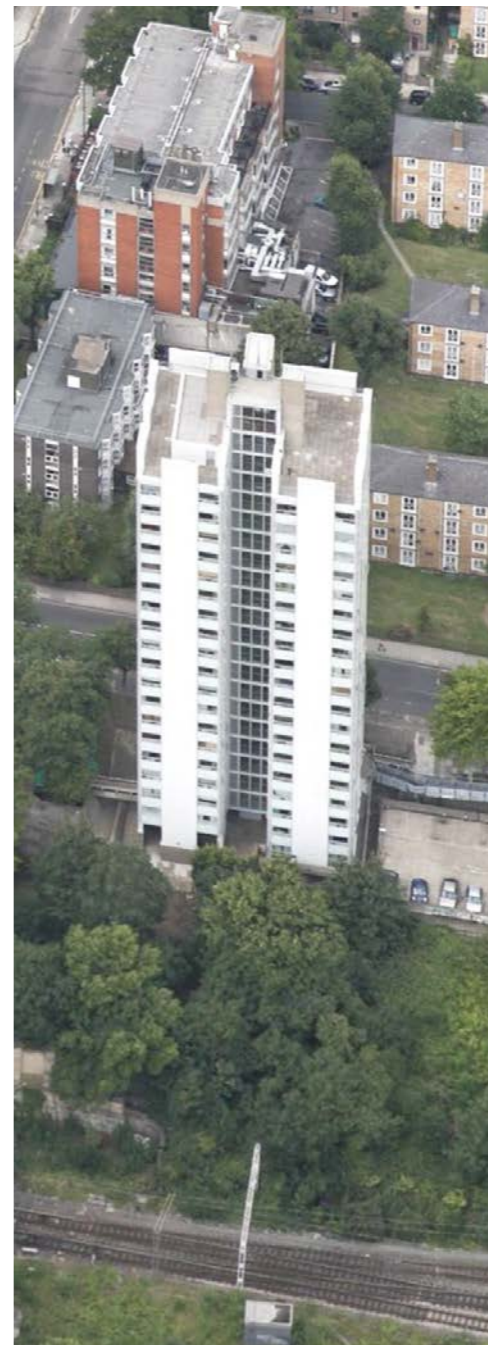
Blashford Tower NW bird's eye view
