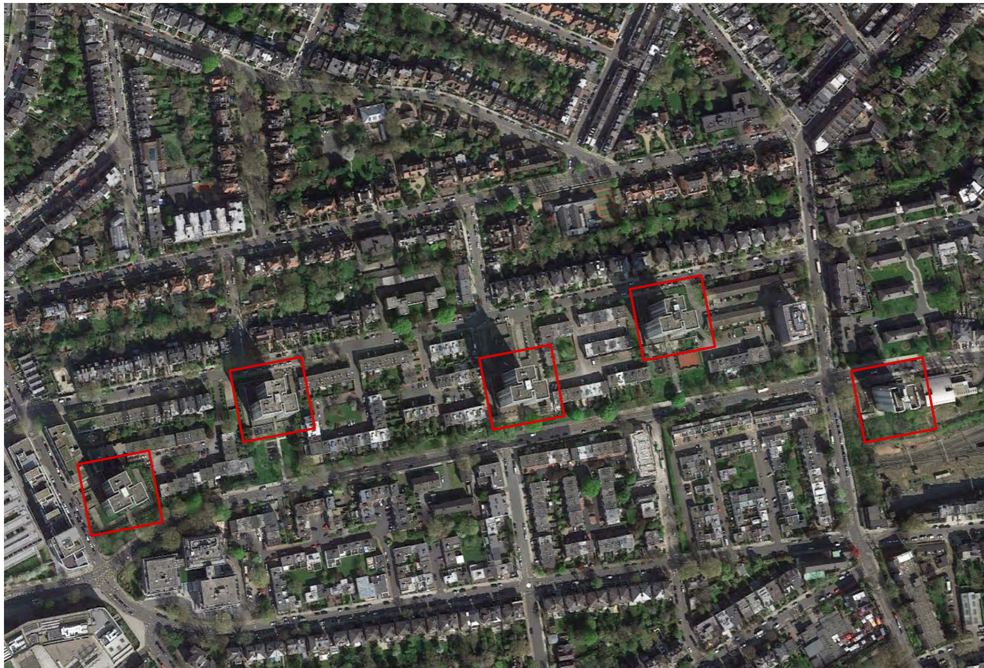
Chalcots Towers Aerial View
