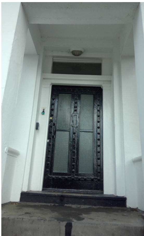
11 Rochester Road – Door detail
