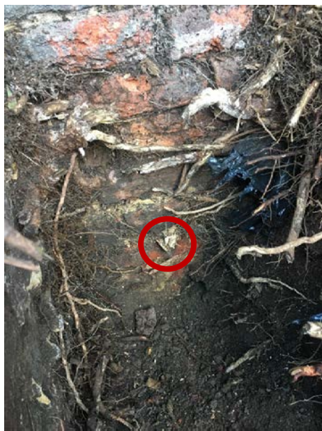
Photo 7 (above right): Taken from above the patio retaining wall with the boundary wall at the top of the photo. T1 lies beyond the boundary wall and the top right-hand corner of the photo. Note the continuation of the boundary wall along the site, essentially forming an underground root barrier for T1. The roots seen in the middle right of the picture in higher quantity are from the mature ivy, the thick stem of which is just visible in the top right edge.
