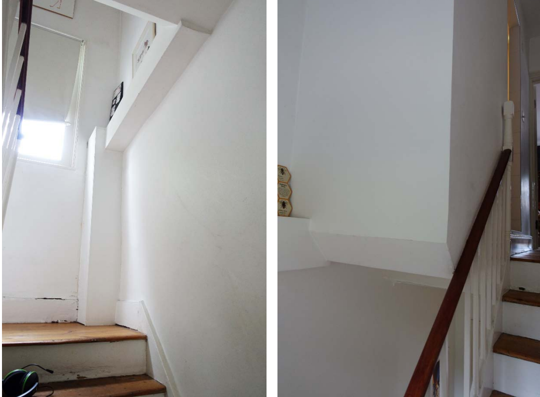
8 – 19. Internal photos of No.133 showing the existing building condition and finishes
