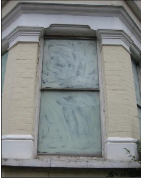
Previous Front Ground Floor Window
