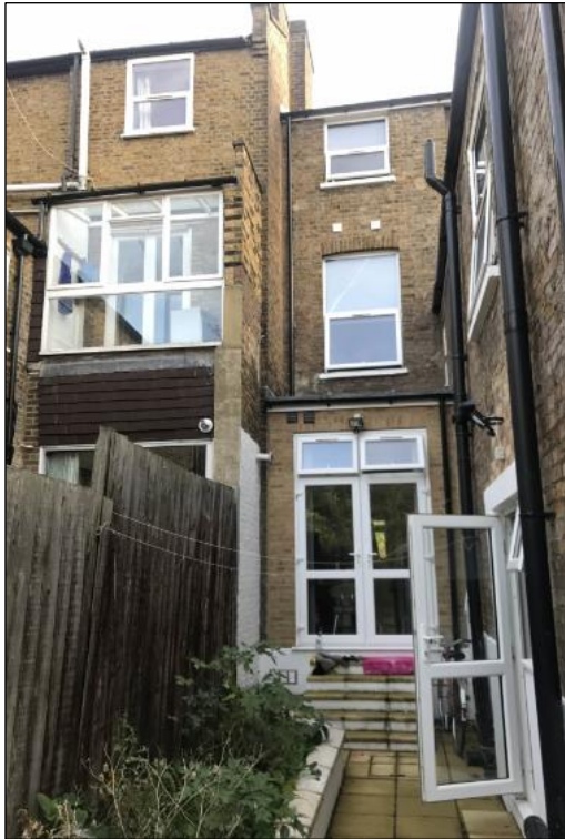
New Windows to the Rear Elevation
