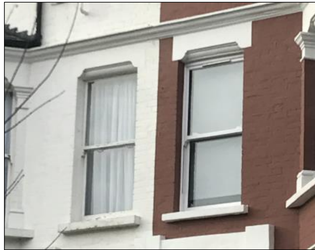
Windows to the Front of No. 5 & No. 7
