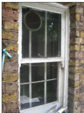
Old Timber Frame Window
