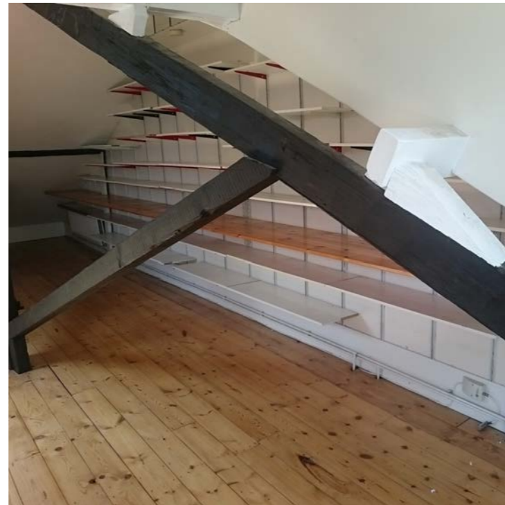
Timber structural beams across Third Floor
