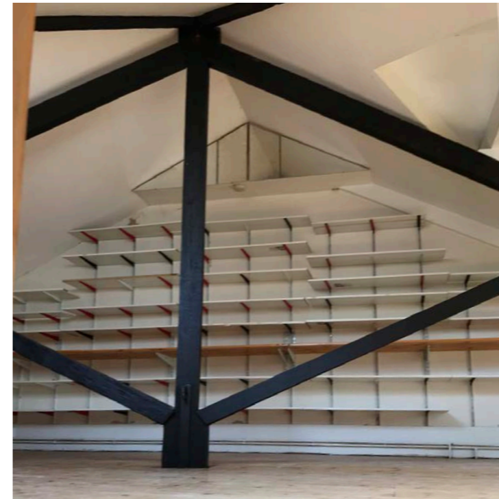
Timber structural beams across Third Floor
