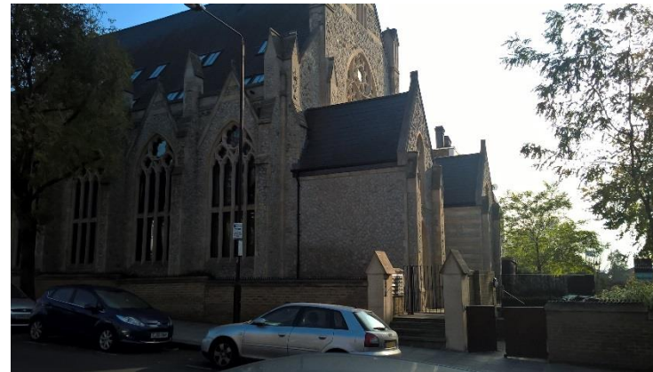
Grove View Apartments – View of Side Elevation
