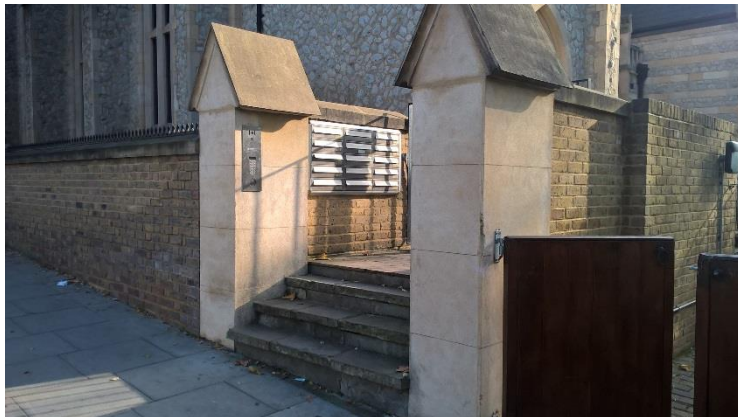
Side entrance from Chetwynd Road
