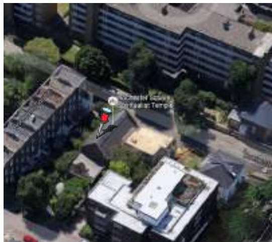
Photo 1 : Bird's eye view of rear elevation
