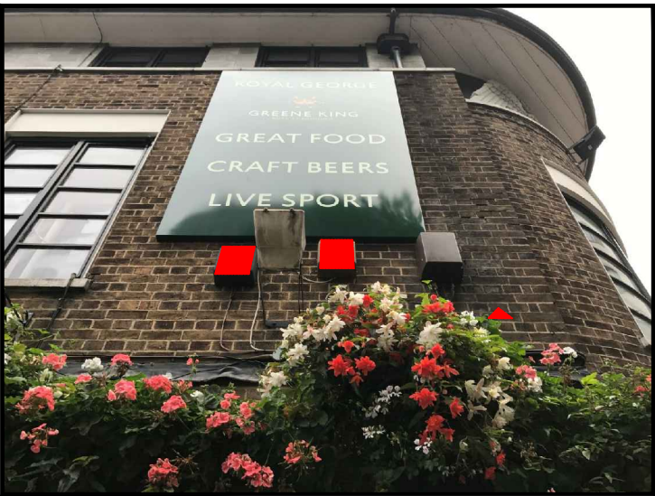
EXISTING ANTENNA A1 & A2 TO BE REPLACED. GPS MODULE (TO BE INSTALLED AT A LATER DATE)
