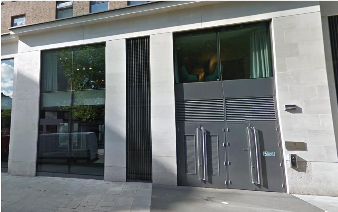
Photo of the East Elevation Louvres located on the ground floor (Bury Place)
