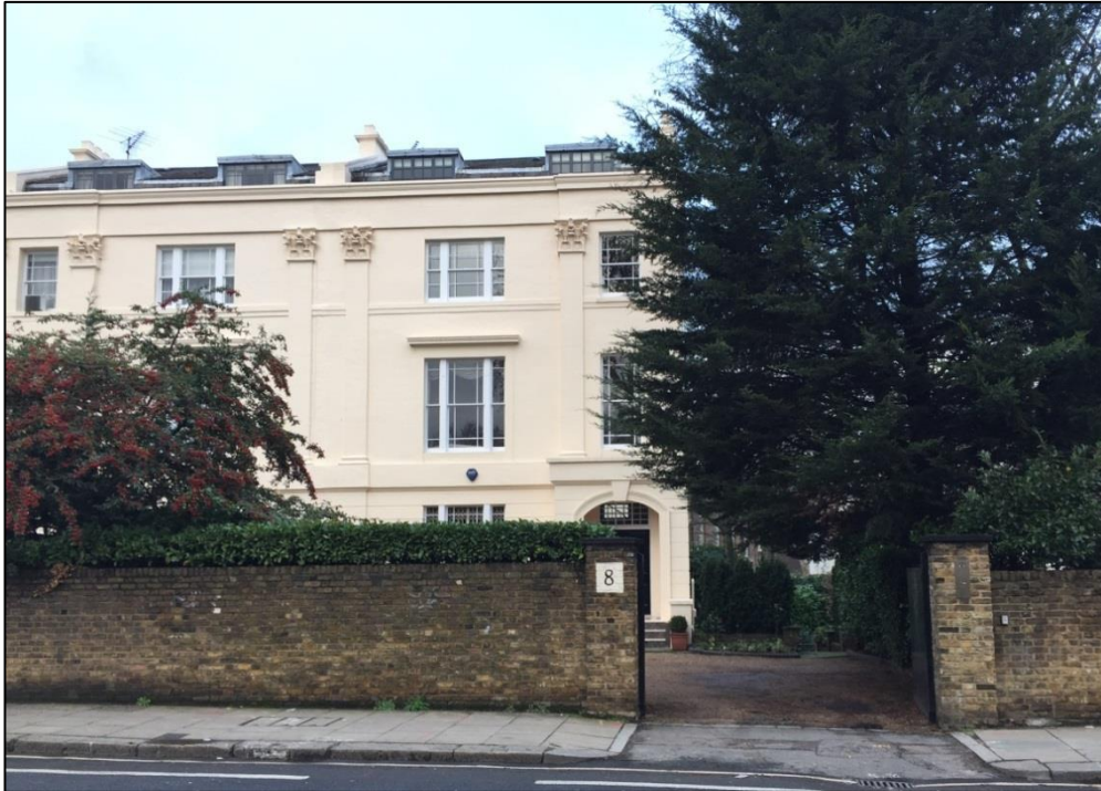
Photograph 2.1 (above): No. 8 Prince Albert Road, Front Façade.
