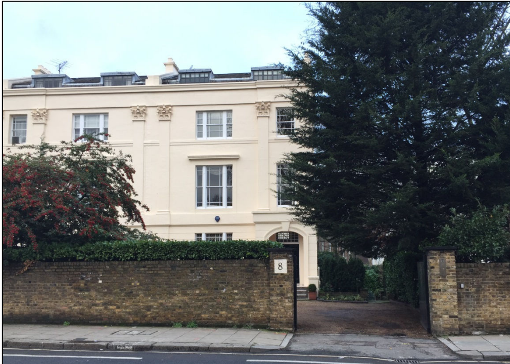
Photograph 2.1 (above): No. 8 Prince Albert Road, Front Façade.
