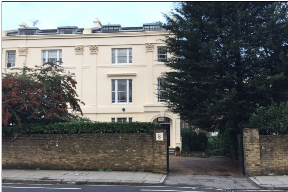
Figure 2.2 No. 8 Prince Albert Road, Front Façade.
