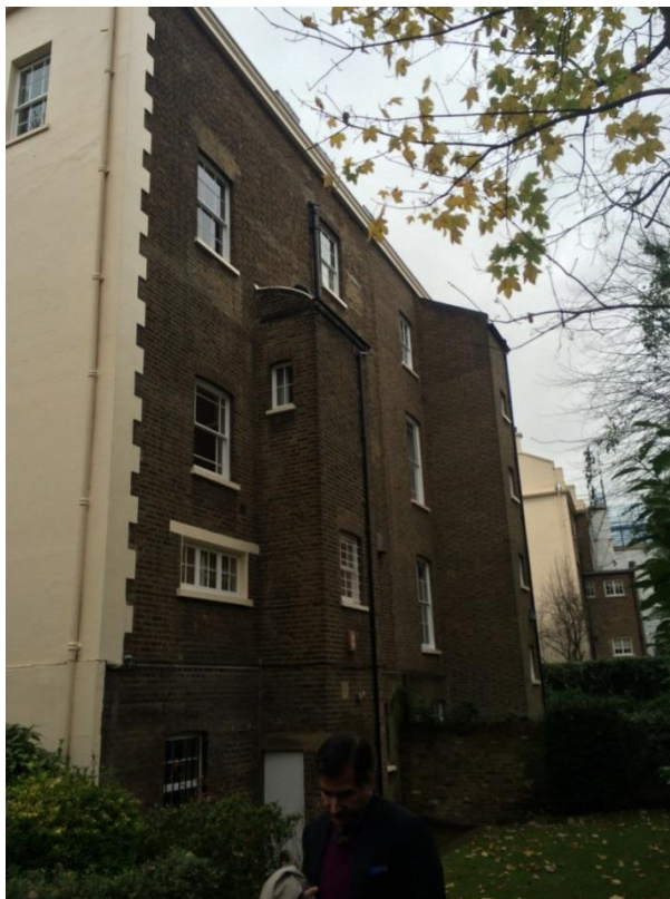
Existing rear facade
