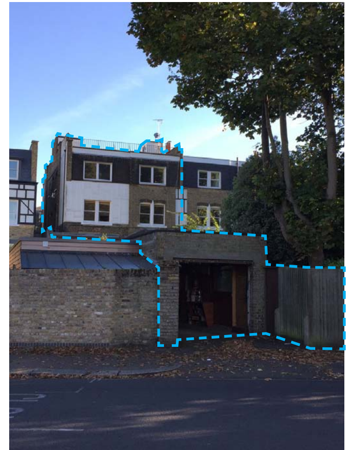
View of the existing property from King Henry's Road - No10 marked in blue
