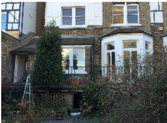
Photograph 3. Existing Rear Elevation
