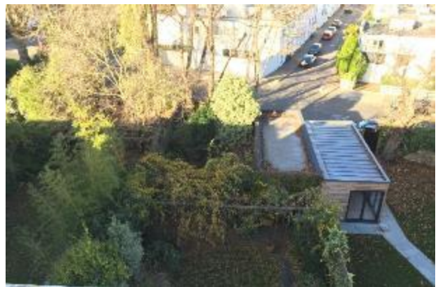
Photograph 4. Existing Rear Garden Building
