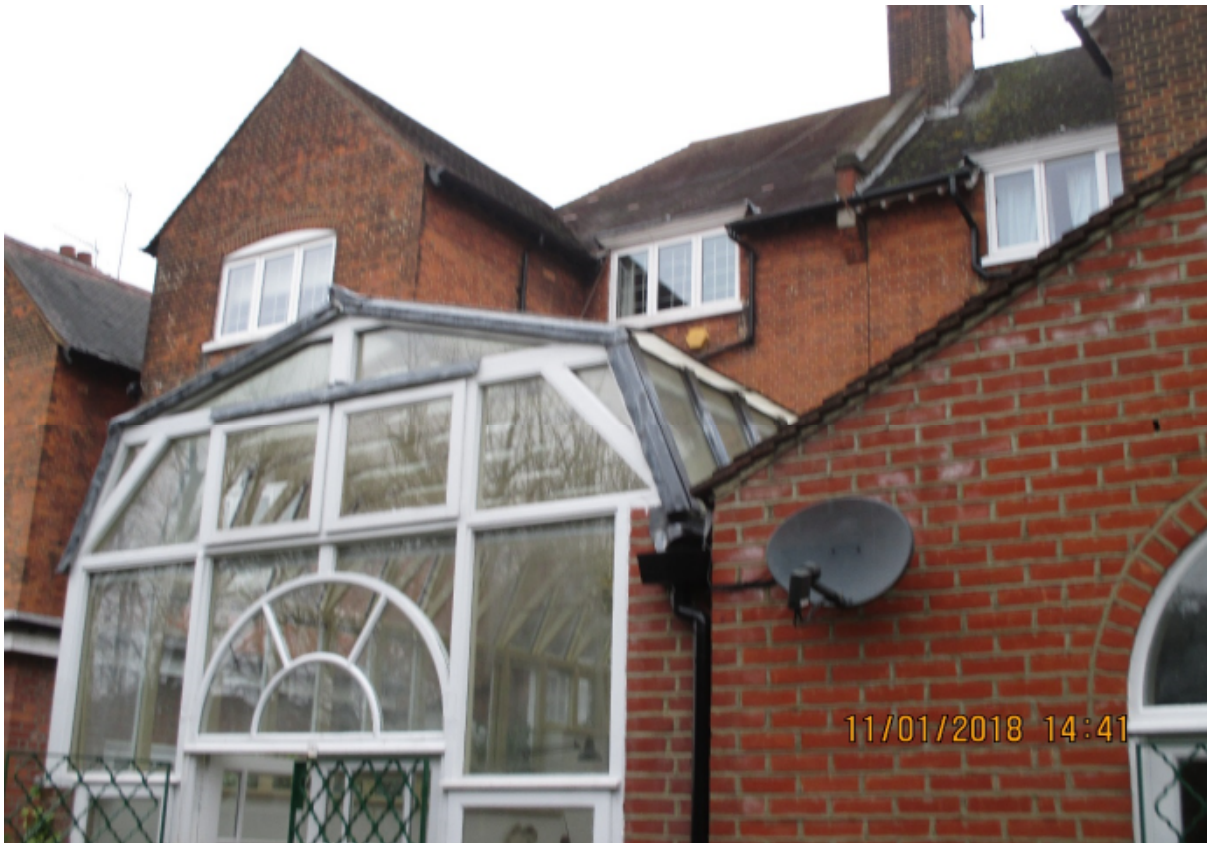
2. Shows part of the conservatory roof
