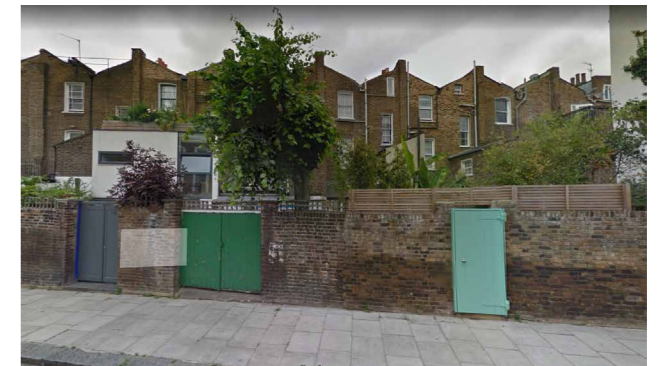
Rear Elevation of Healey Street From Grafton Crescent
