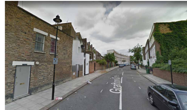
Rear elevation from Grafton Crescent
