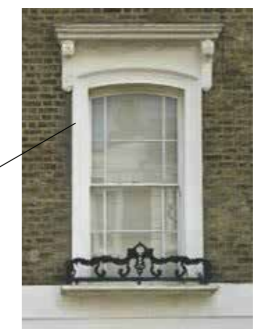
Existing rendered surround windows
