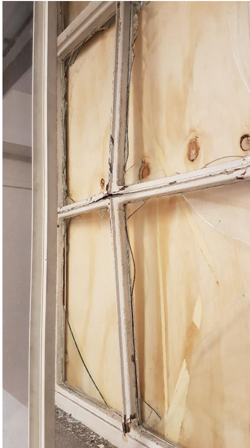
Steel Casement Window Bent Inwards
