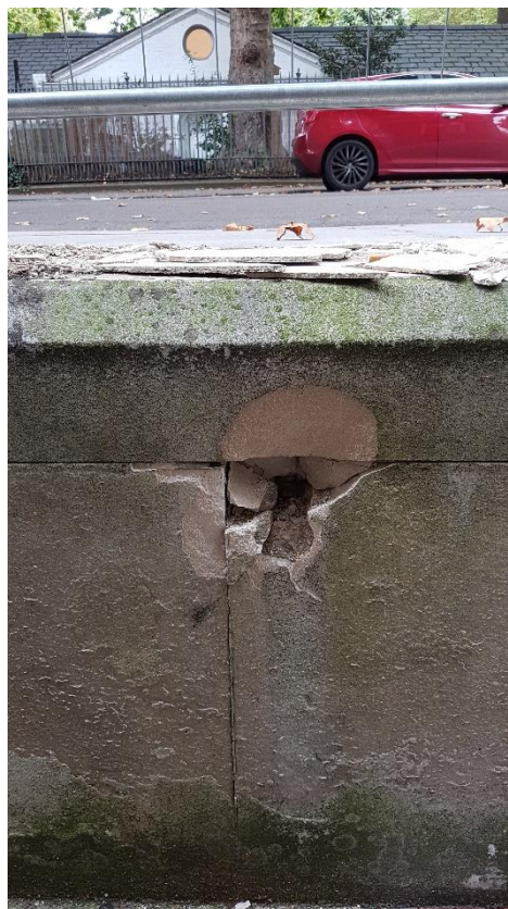
Damaged Wall Where Post Has Pulled Out
