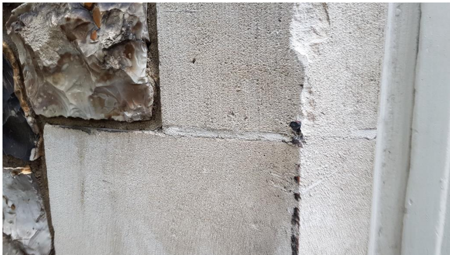
Left Hand Reveal. Spalled Stone and Paint Staining
