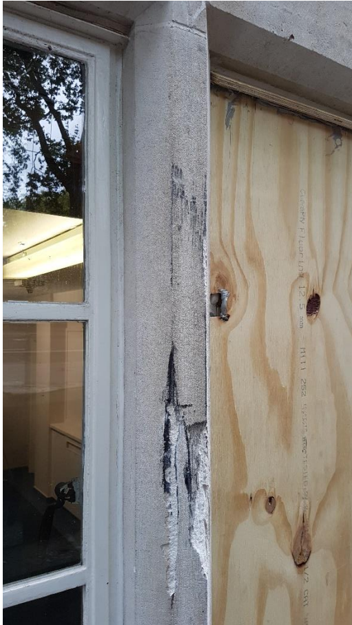
Left Hand Mullion. Spalled Stone and Staining
