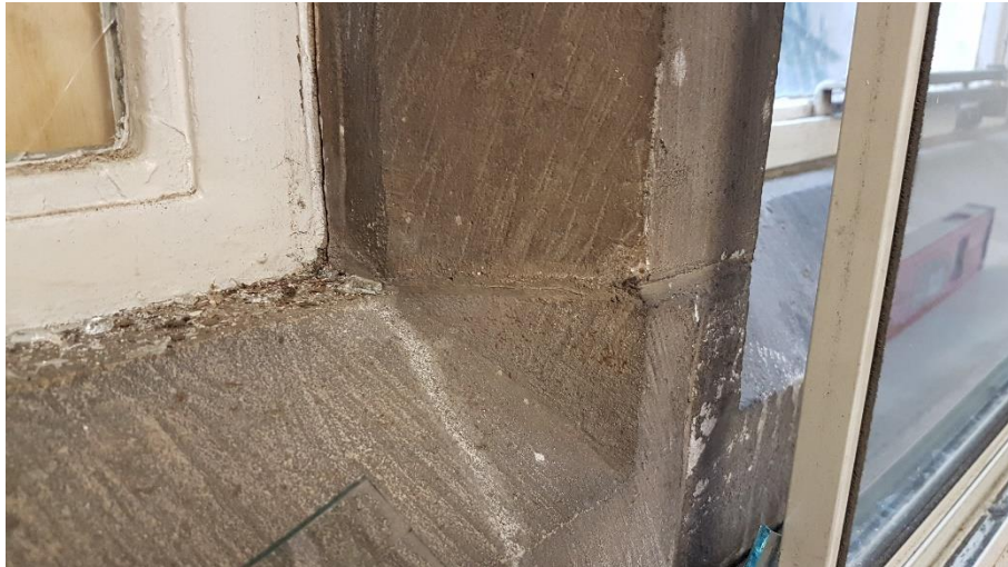
Joint at Bottom of Mullion – Internal
