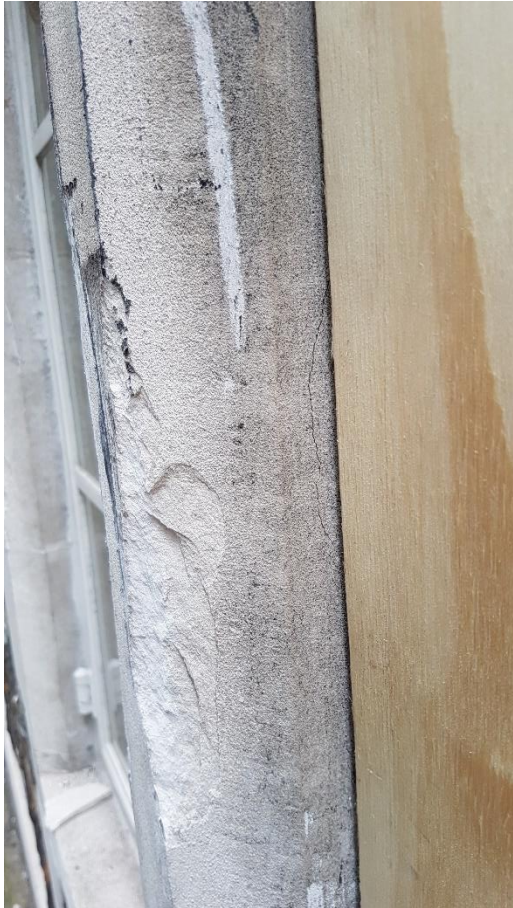
Crack to RHS of Mullion - External
