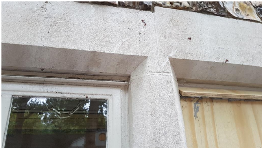
Joint at Top of Mullion - External
