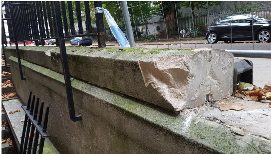
Damaged Coping – Note the Support Dowel in the Lower Wall
