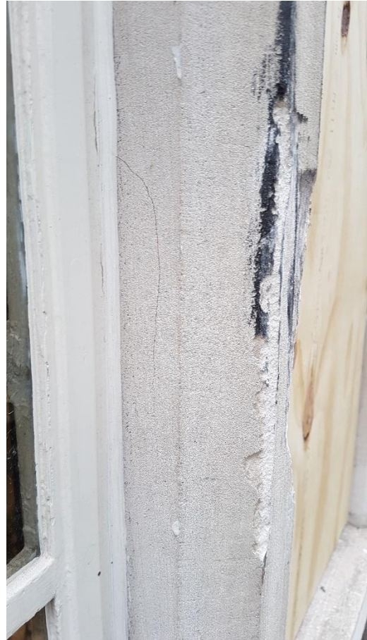
Crack to LHS of Mullion – External
