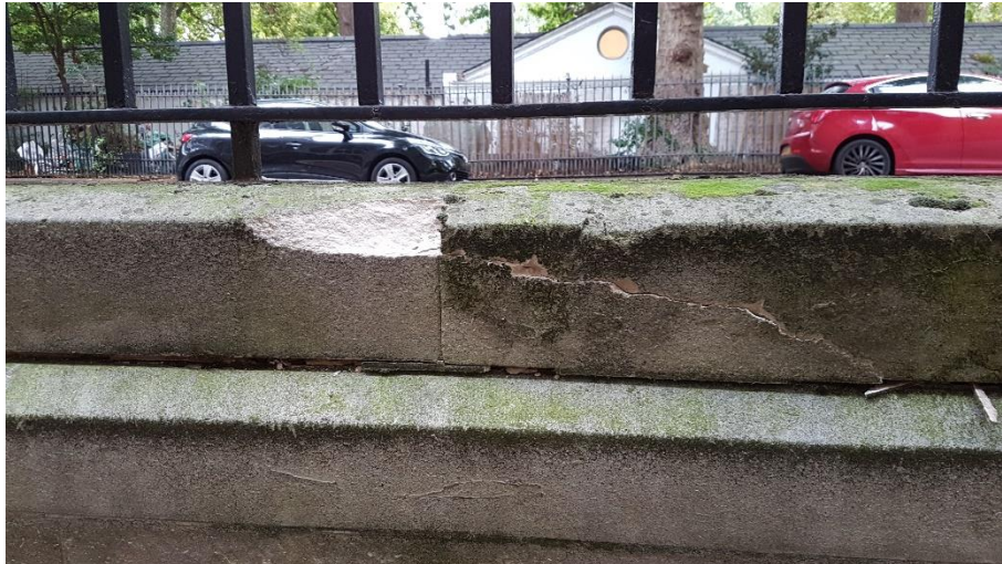
Cracked and Damaged Coping
