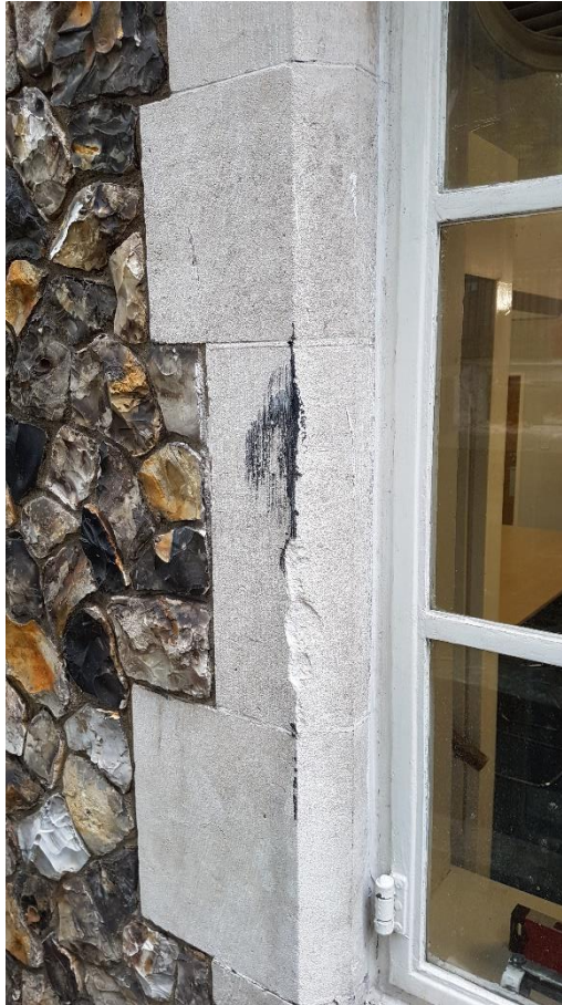
Left Hand Reveal. Spalled Stone and Paint Staining
