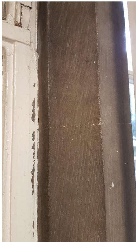
Crack to Mullion - Internal
