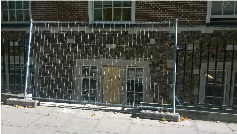
Typical Elevation Showing Flint Wall and Portland Stone Windows
