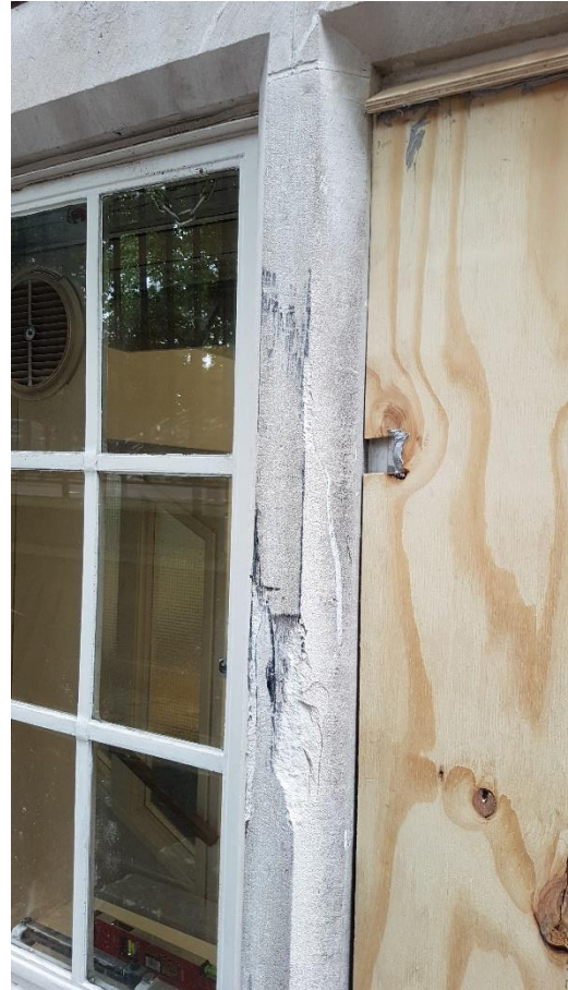
Left Hand Mullion. Spalled Stone and Staining
