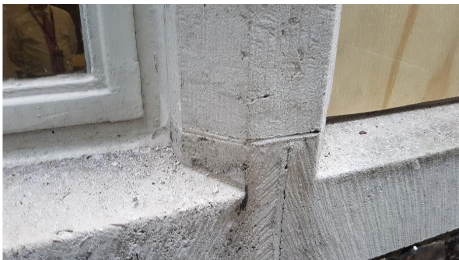
Joint at Bottom of Mullion – External
