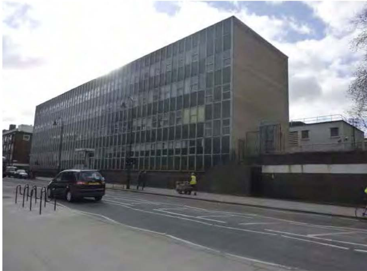
View of the site on Guilford Street looking south east
