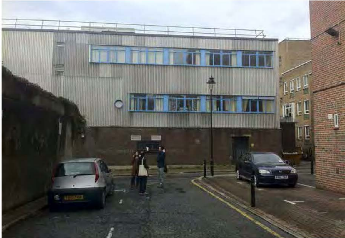
Rear of the site on Millman Mews
