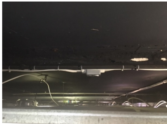
Fig. 12 - Existing concrete block and beam ceiling above suspended ceiling tiles.
