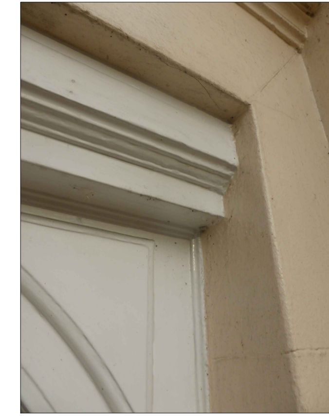
Existing fan light: No10 head
