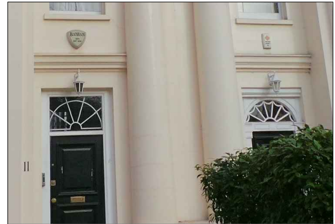
Existing front doors: No 11 on left, No 10 on right.
