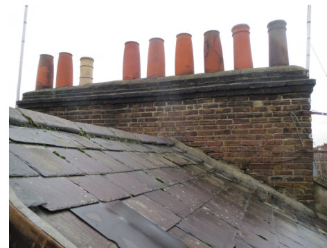
ORIGINAL SLATES and ridge tiles
