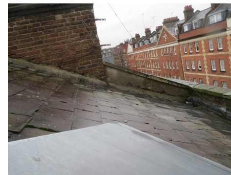
missing slates and intrusive services
