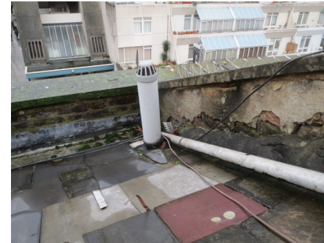
missing slates and intrusive services
