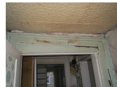
door fitted with infill panel due to deflection
