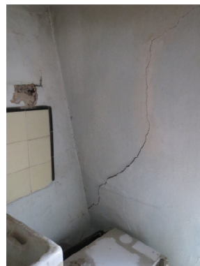
raking crack to mansard roof at rear
