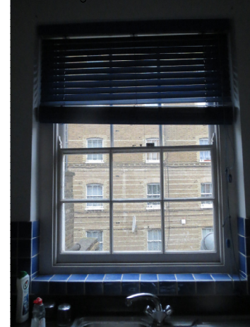
modern replacement window
