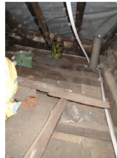
PARAPET GUTTER BOARD IN CRITICAL CONDITION
