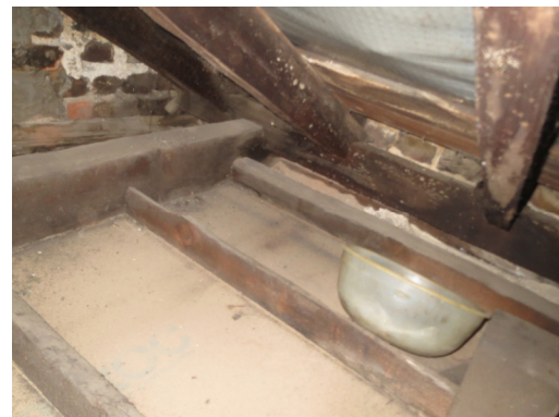
PARAPET GUTTER BOARD IN CRITICAL CONDITION
