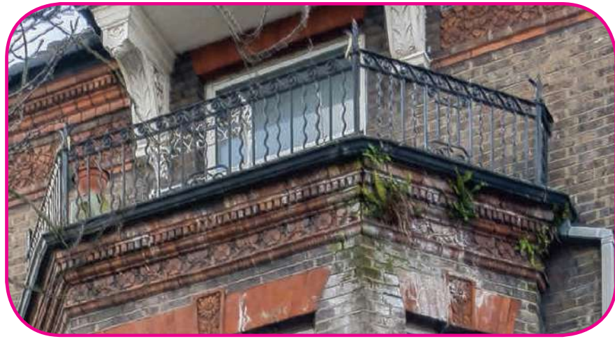
DETAIL 2 REFERENCE IMAGE - PICTURE OF EXISTING RAILING TO FRONT BALCONY
