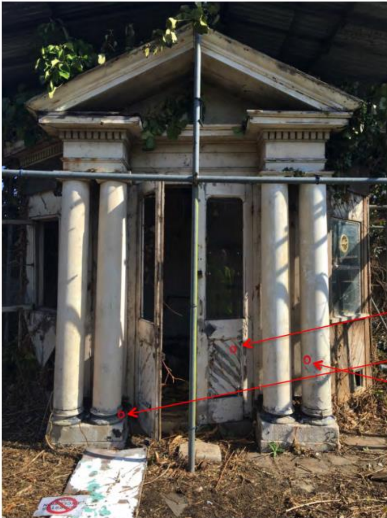
Figure 1: Portico façade of the Summer House
