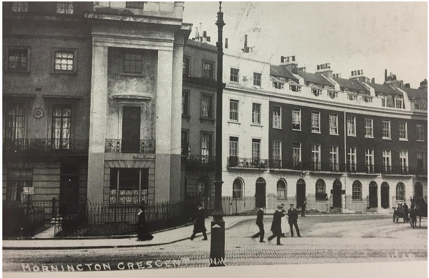
Fig 13 A view of Mornington Crescent from Hampstead Road c.1905 – note the original bottle balustrade at mansard level which has already been removed at nos. 7 and 8 as well as the original gothic ground floor windows at nos. 5, 6 and 7.
