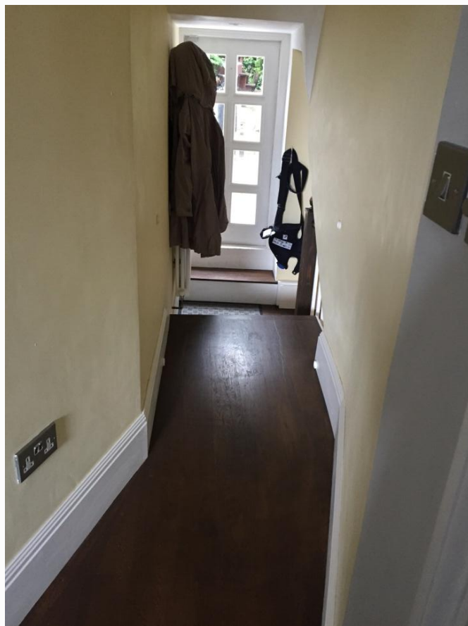
Fig 28 The internal corridor to the flat at ground floor level.
