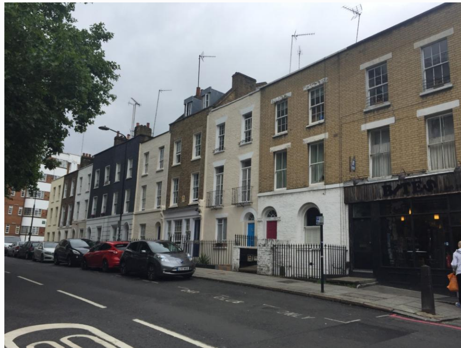
Fig 8 Nos.37-46 Mornington Crescent.
