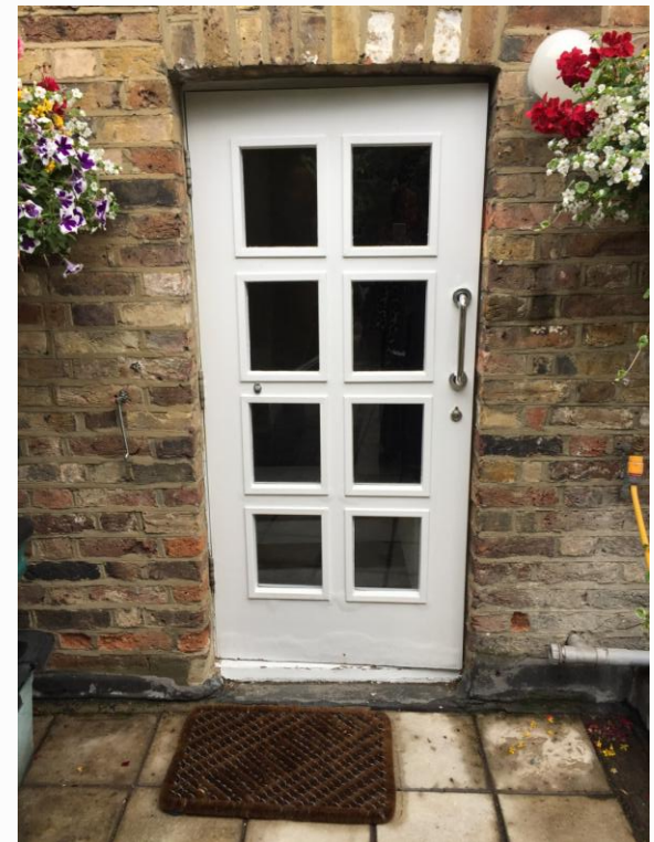
Fig 34 The modern door within the rear elevation.
