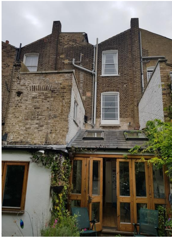
Existing Rear View
