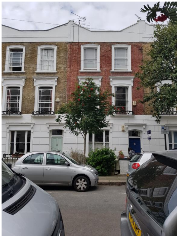
Existing Front View
