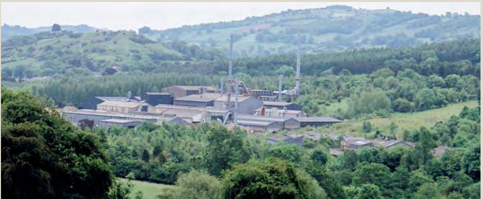
Operated by HJ Enthoven and Sons, Europe's largest Lead recycling facility in the heart of the Derbyshire Dales is the key to BLM's strategy to producing a fully recycled range of Lead products.
