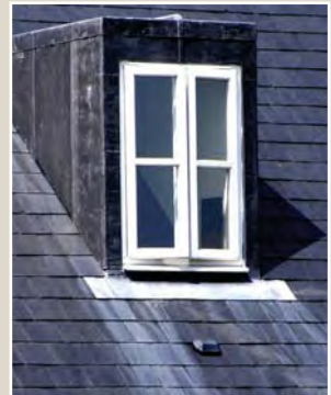
Carbonate staining when Patination Oil is not used.
