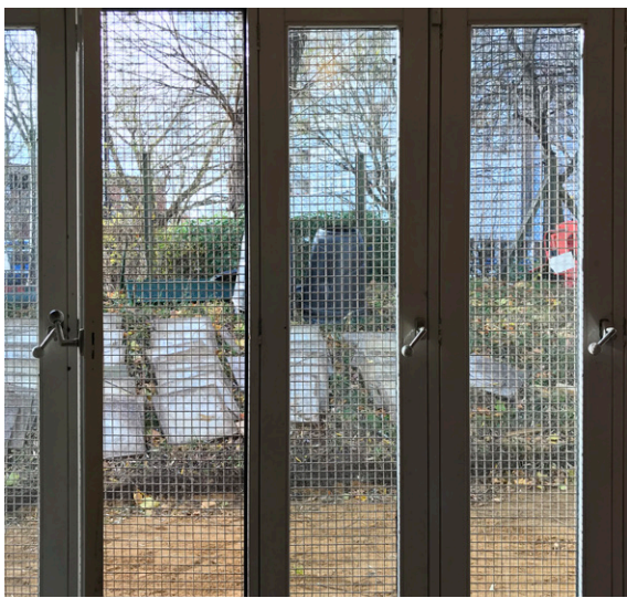
Fig. 4. Glazed doors to rear garden.
