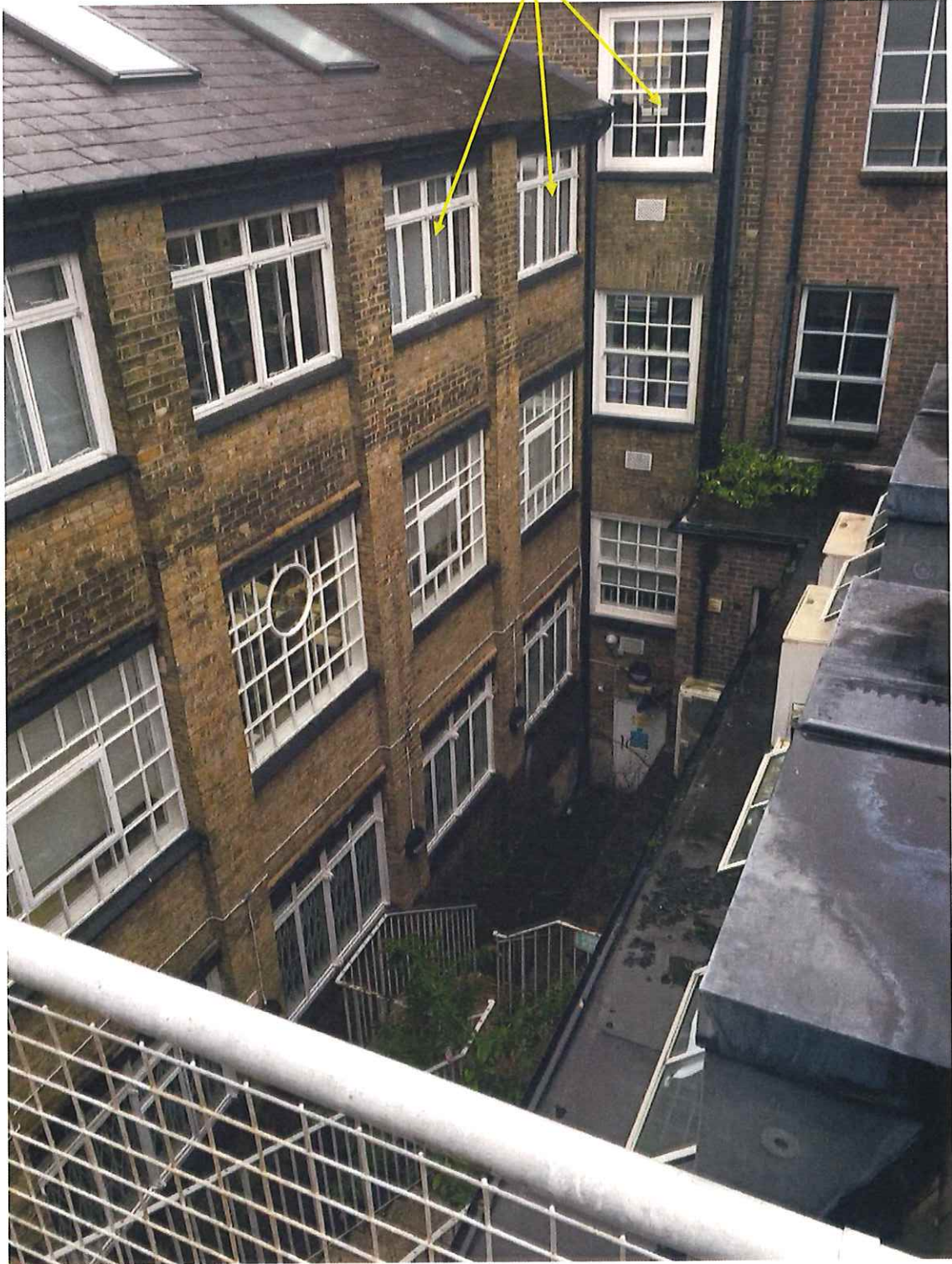
Photo H – Lightwell on Left Hand Side of Second Floor Roof
